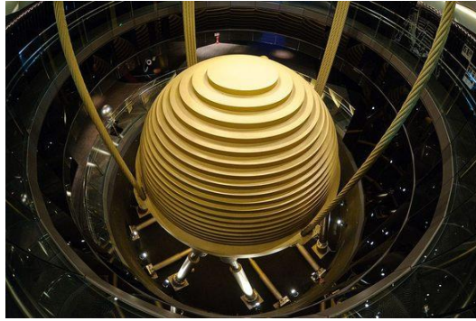
Figure 1.6: Tuned mass damper
