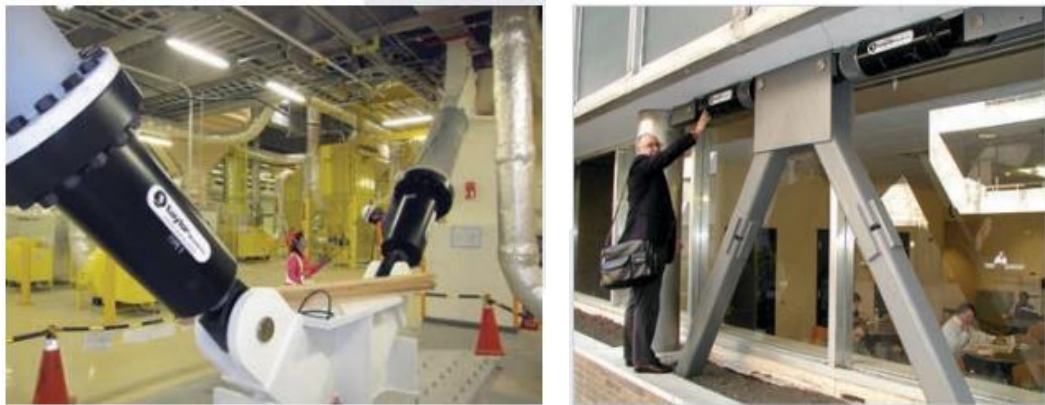
Figure 1.4: Fluid viscous damper ( taken from Taylor Devices Inc. catalogue )
