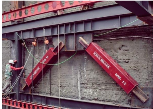
Figure 1.5: Buckling-restrained braces ( taken from Vira Brace Inc. )
